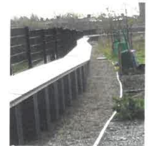
Example sheet pile wall with timber coping
