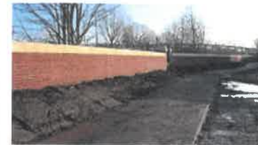
Example sheet pile wall with timber coping
